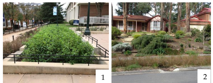
Figure 1: A bio retention system on the University of Virginia Grounds intercepts storm water through screened inlets, thereby reducing, slowing and improving water quality. Most of the intercepted runoff is consumed by vegetation, percolates into groundwater, or is temporarily stored and then slowly released [7] .
